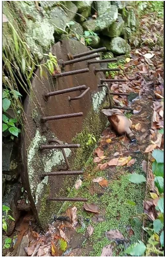
30" pipe capped off
