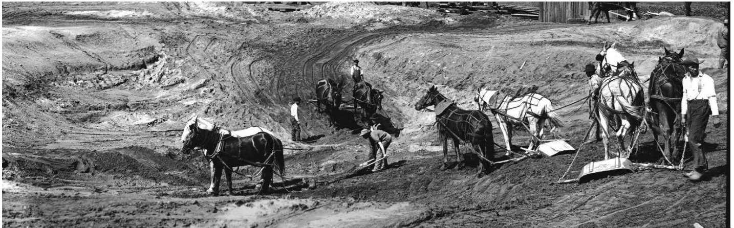
Picture shows how they moved dirt prior to the heavy motorized equipment we have today. We believe this is how they dug the canal and made the 900’ Berm along the Canal in 1863.
