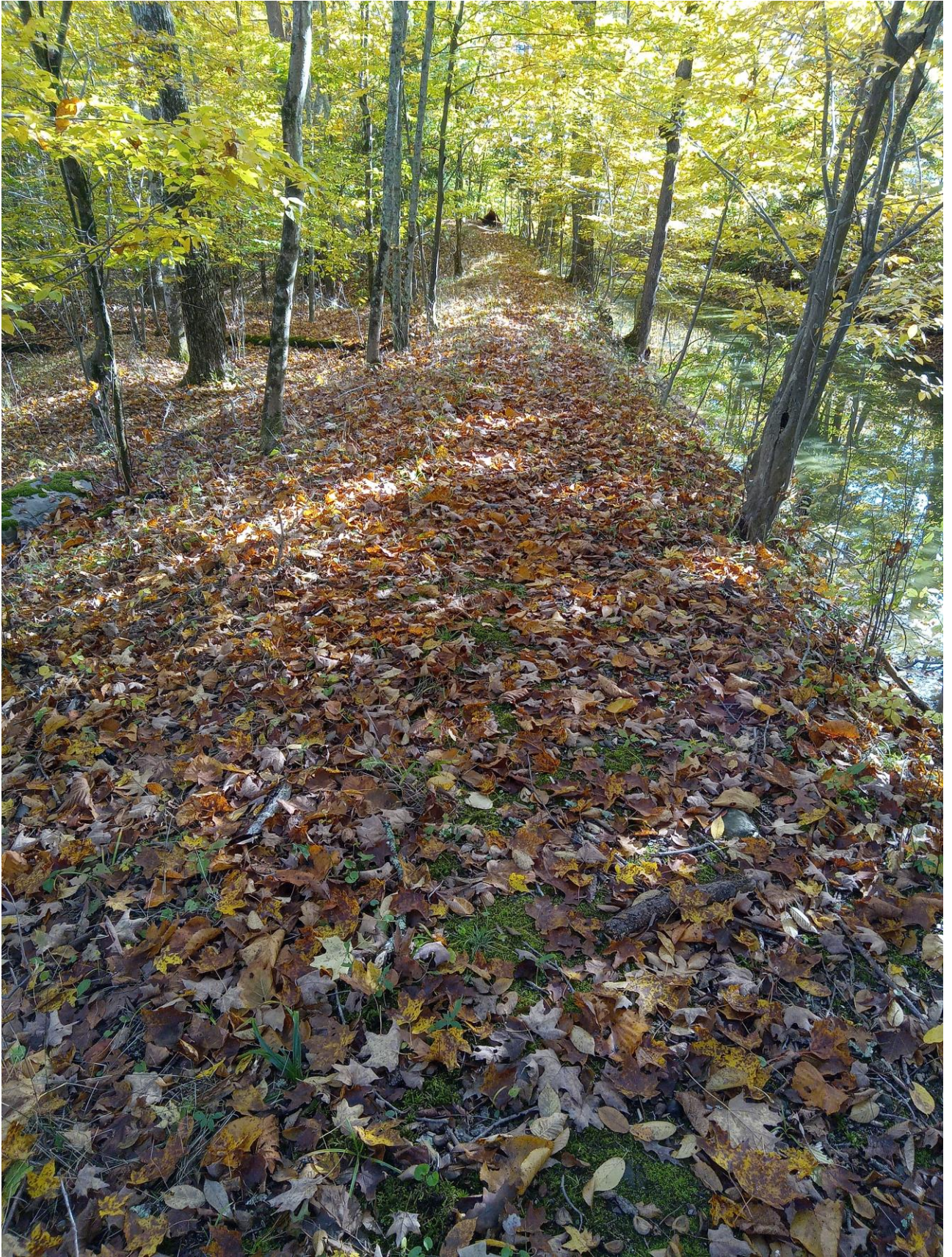
Berm after the flood, canal to right.
