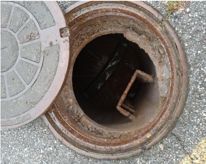
Sewer manhole at least 10' deep.
