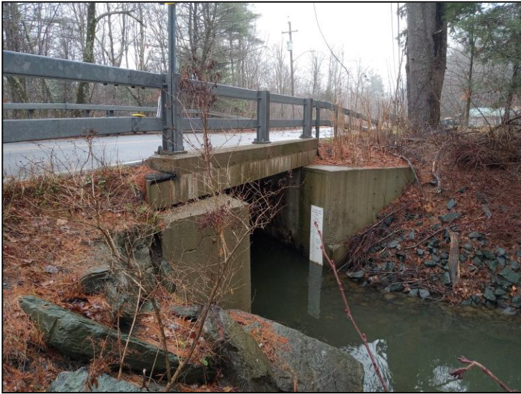
Lake side of Spillway
