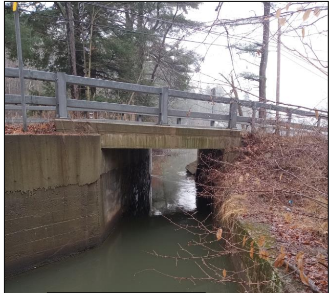
Canal side of Spillway
